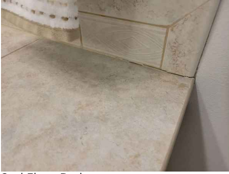
2nd Floor Bathroom
