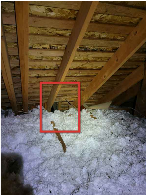
Front Lower attic
