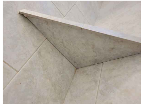
2nd Floor Bathroom
