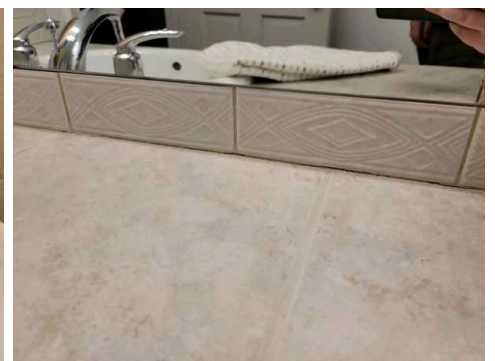
2nd Floor Bathroom
