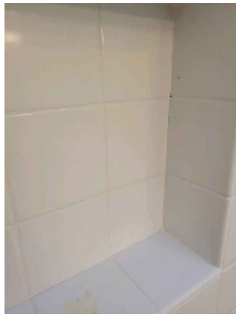
2nd Floor Bedroom Bathroom
