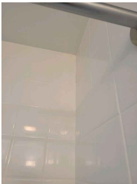
2nd Floor Bedroom Bathroom
