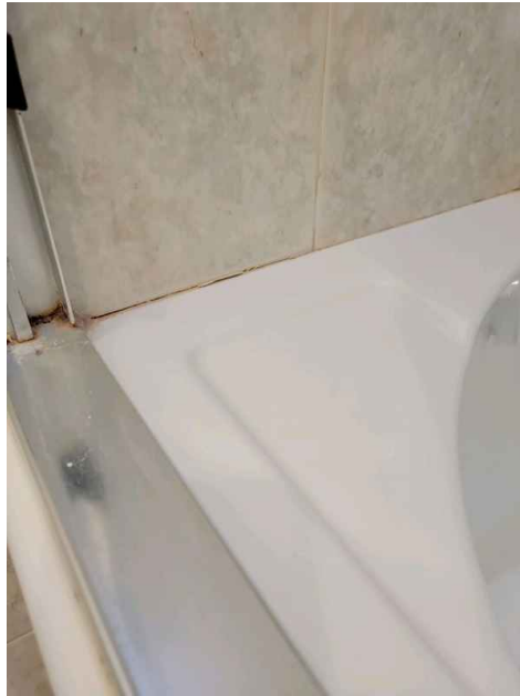
2nd Floor Bathroom
