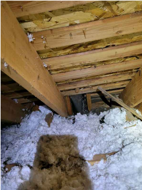
Front Lower attic
