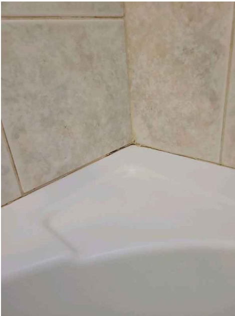
2nd Floor Bathroom
