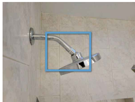
2nd Floor Bathroom
