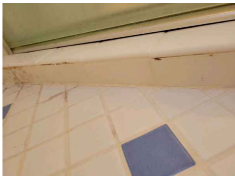
2nd Floor Bedroom Bathroom
