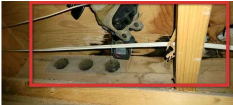
Partial Attic at Front Game Room, Elevated moisture reading
