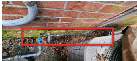
Current Exterior AC Unit Not Connected to New Furnace
