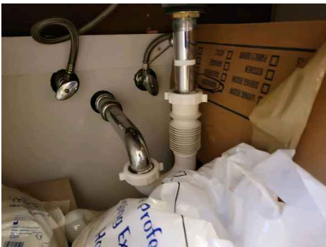
1st Floor Bathroom
